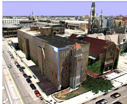
Community Correction Center
