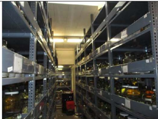
Artifact Storage on Upper Floors
