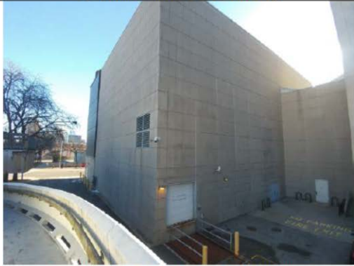
Southeast at Dock Area of DW Building
