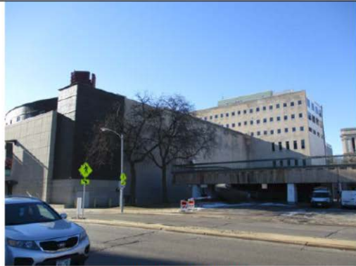
Southwest at DW Building
