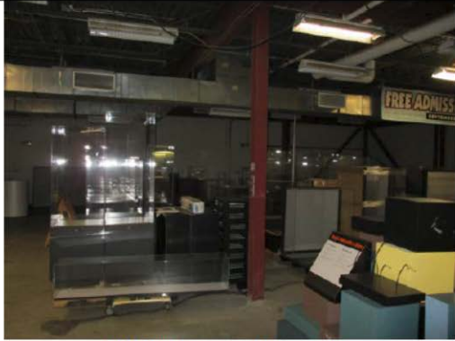
DW Building – Shell Condition
