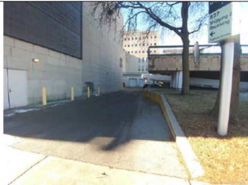
Access to Dock Facilities from N. James Lovell St.
