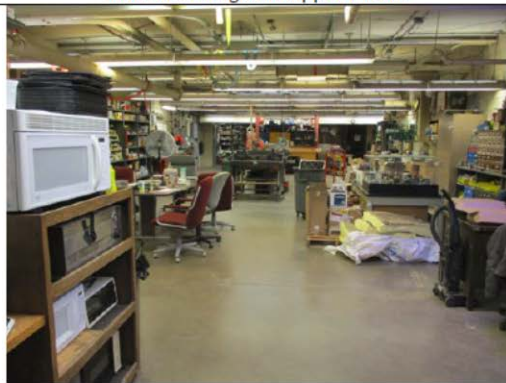
Mechanical/Maintenance in Basement of MPM
