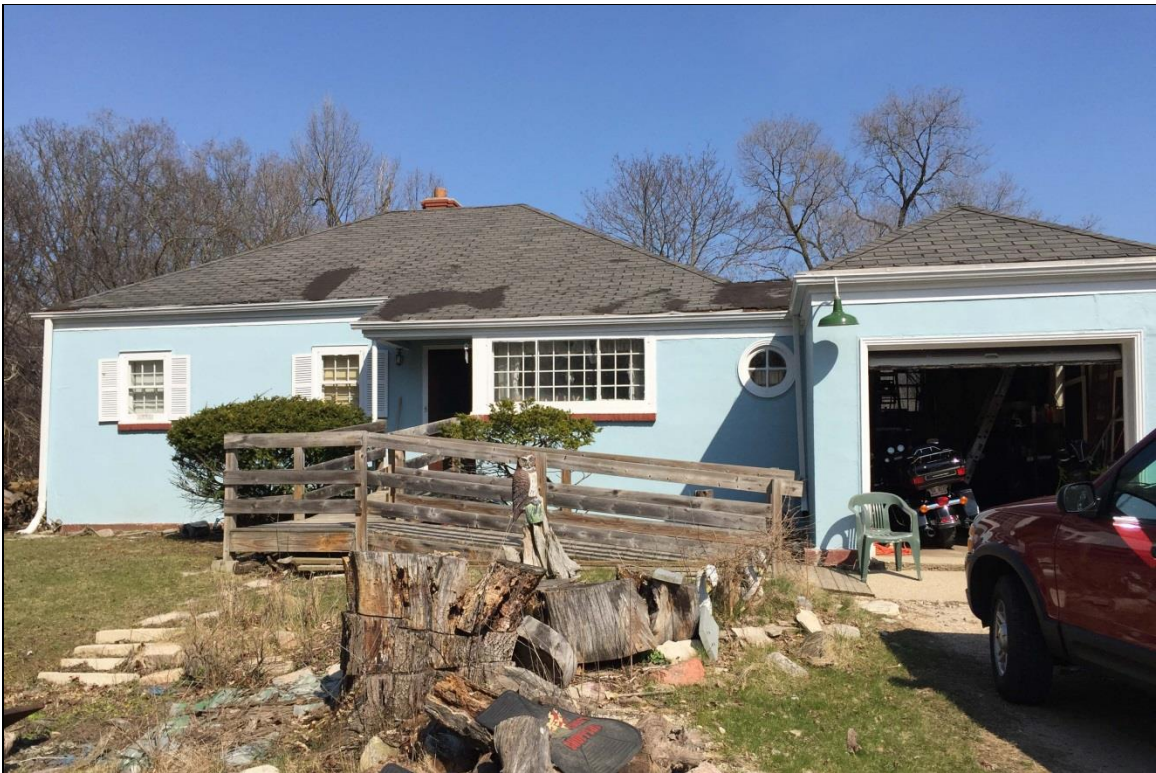
Front Of Subject Property
