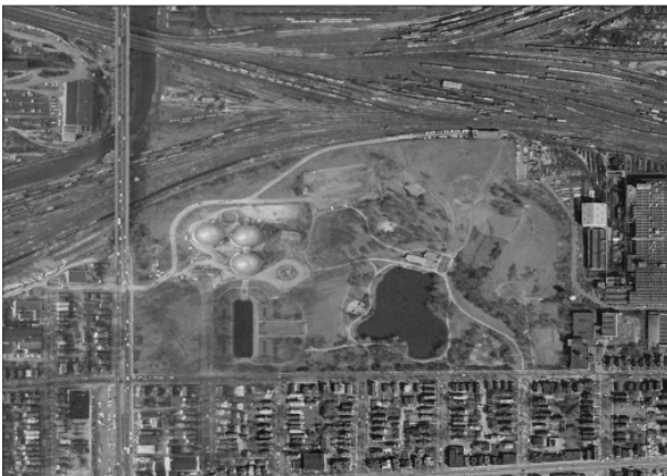
Domes under Construction, 1963
