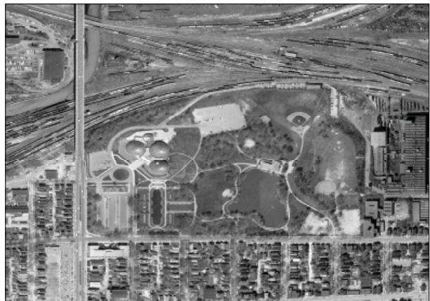
Construction Complete on the Domes, 1967
