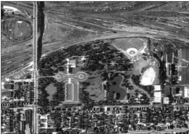
Original Victorian Conservatory, 1937
