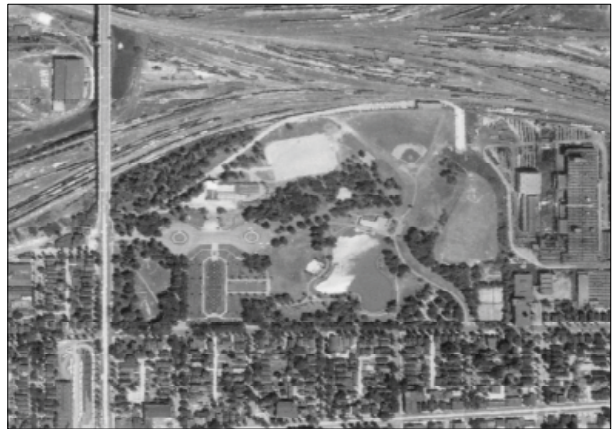
Demolition of Victorian Conservatory, 1956
