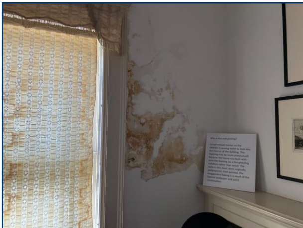
Water leak cause by comprised mortar (description per sign)
