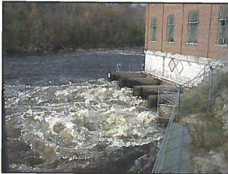
Grandfather Falls Dam along the Wisconsin River
