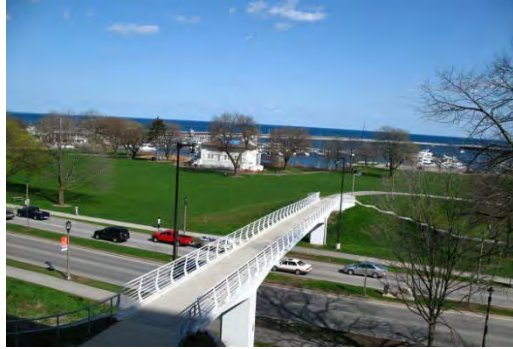
Brady Street Bridge
