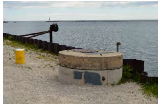
Sewer structure and mooring dolphin
