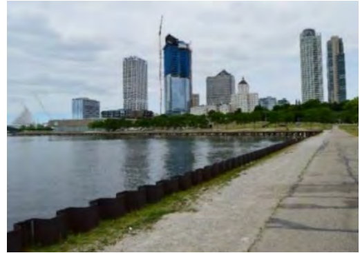
Sheet pile and asphalt trail
