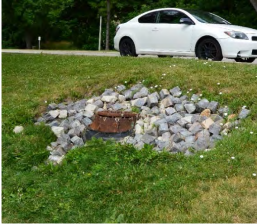
Storm Sewer Outfall along LMD
