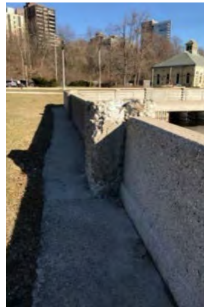
Flushing Tunnel inlet wall at north end
