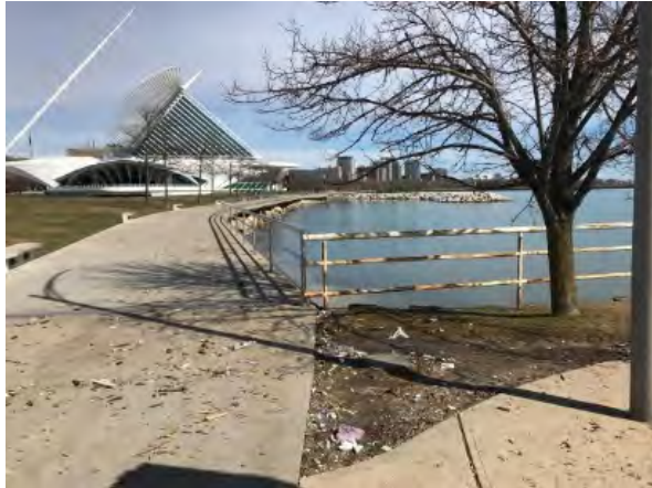
Square corner collects debris
