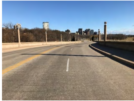
Mason Street Bridge Ramp looking North
