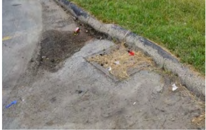
Parking lot inlet
