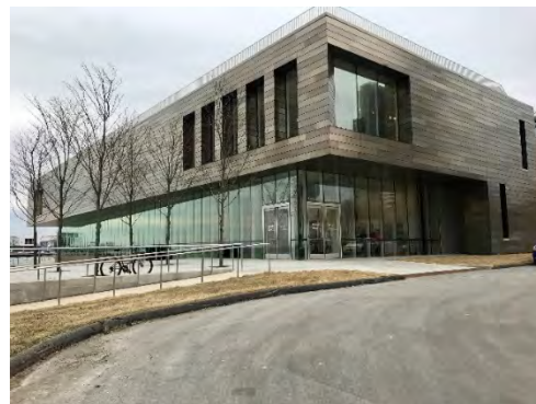
New MAM East Addition Entrance
