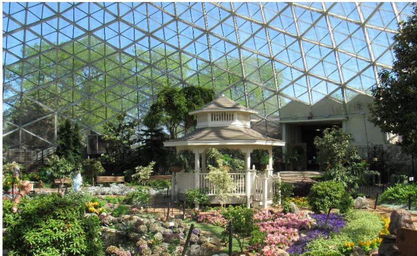
Source: Floral Show Dome picture taken by the Milwaukee County Audit Services Division
