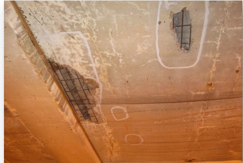
Upper Left: South Kilbourn Tunnel ceiling at voided slab, netting installed in the outline in 2010 to catch falling concrete debris.
