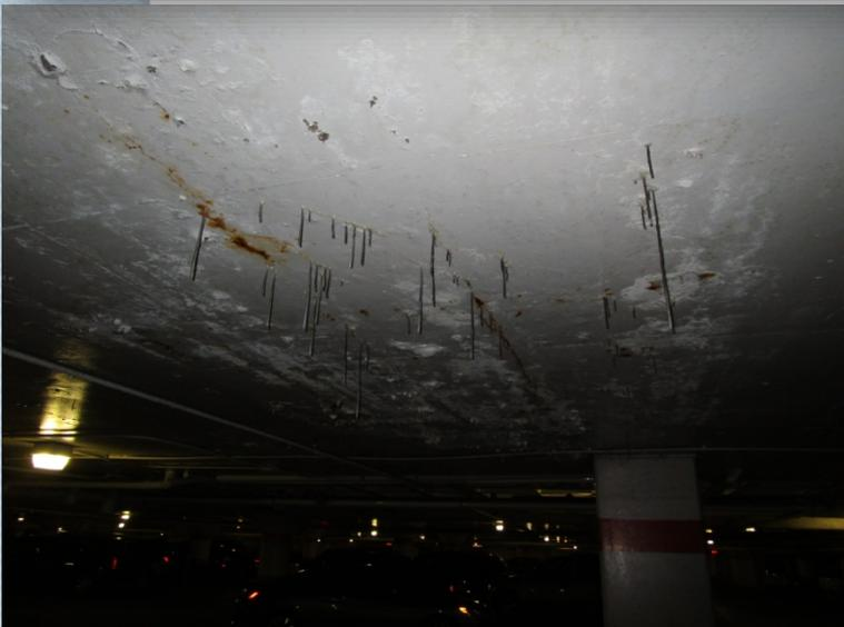
Lower Left: Parking Garage ceiling has large cracks and leaking water.
