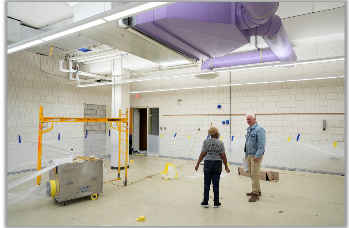
Phase 1 Clinton Rose Senior Center Facility Upgrades Construction
