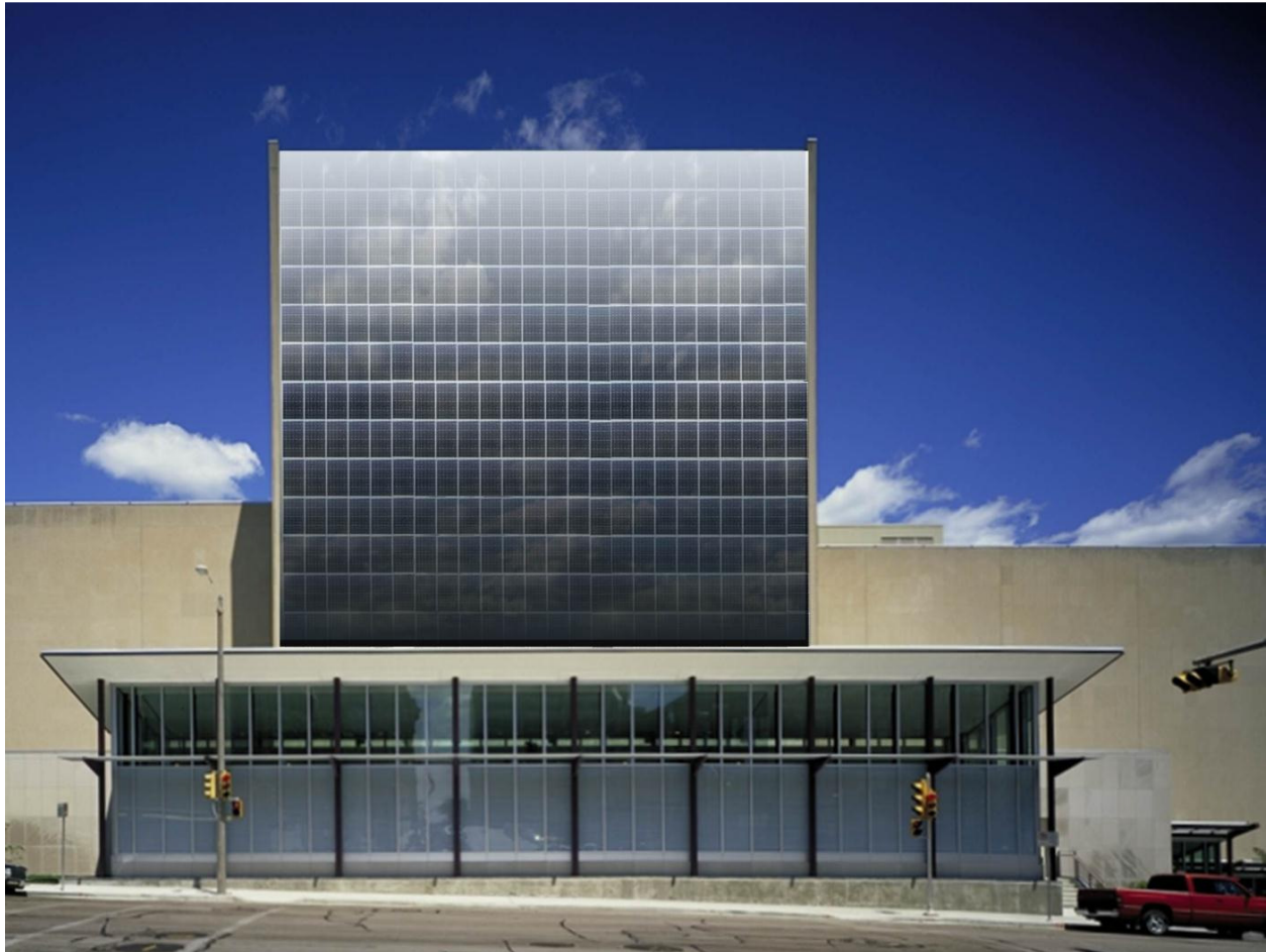
Milwaukee Public Museum with PV Array installed.
