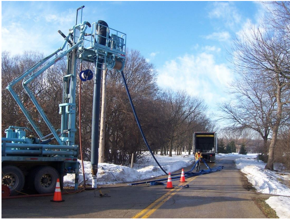
Installing CIPP pipe Liner in Brown Deer Park
