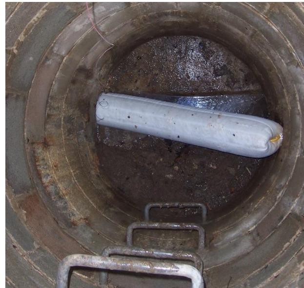
Installing CIPP pipe Liner in Brown Deer Park
