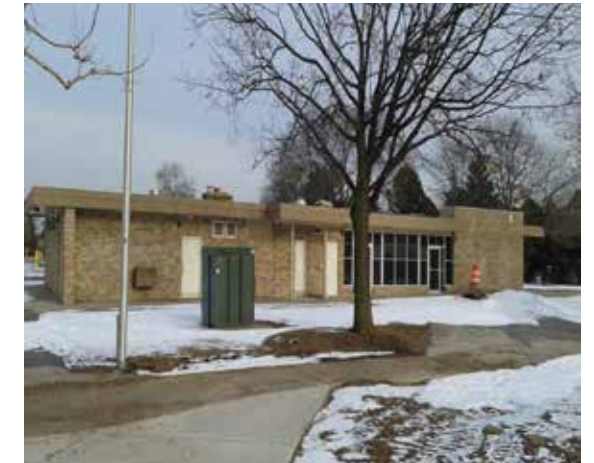
View of existing park bathhouse looking east
