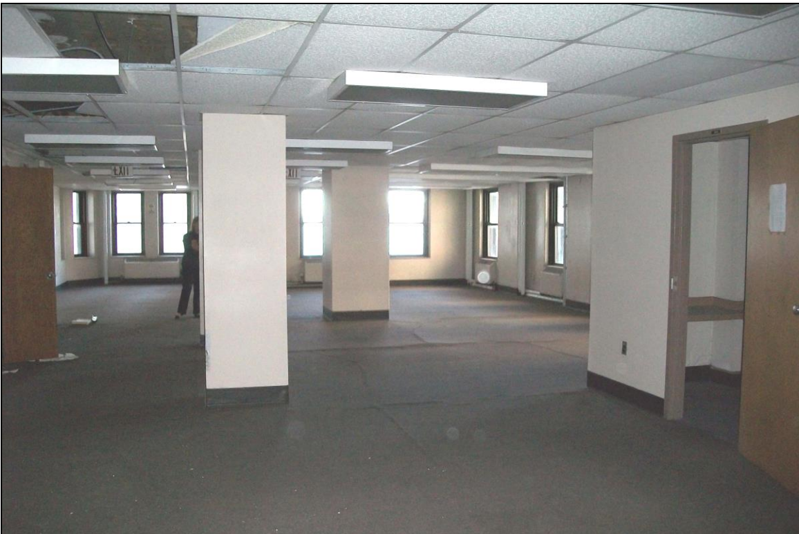
Typical Interior Finish
