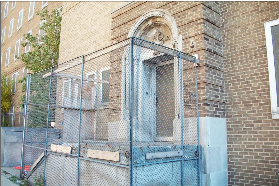
Main Entrance On N. 10 th Street
