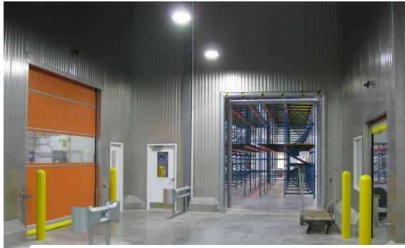
Patrick Cudahy Storage Expansion – 55,000 sf
