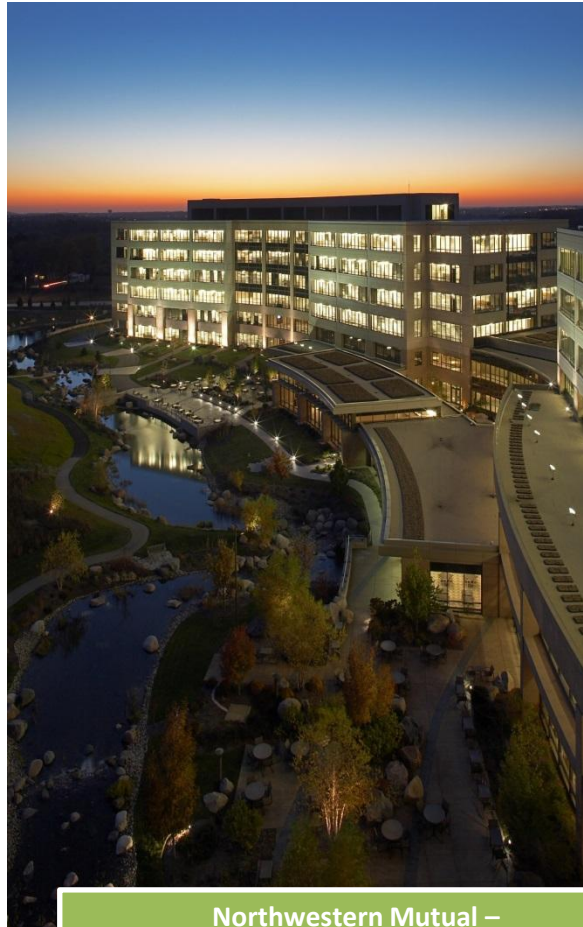
Northwestern Mutual – Phase I & II - 950,000 sf total
