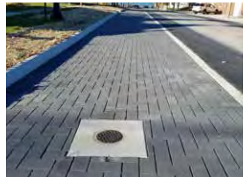
Examples of green infrastructure: rain garden protecting a high-quality woodland (top) and pervious pavement preventing runoff to a beach (bottom).
